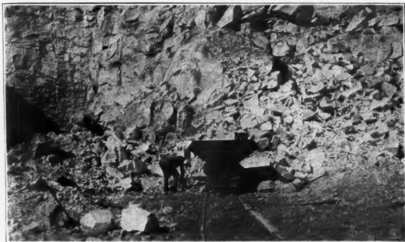
Loading Dump Car in Quarry.
